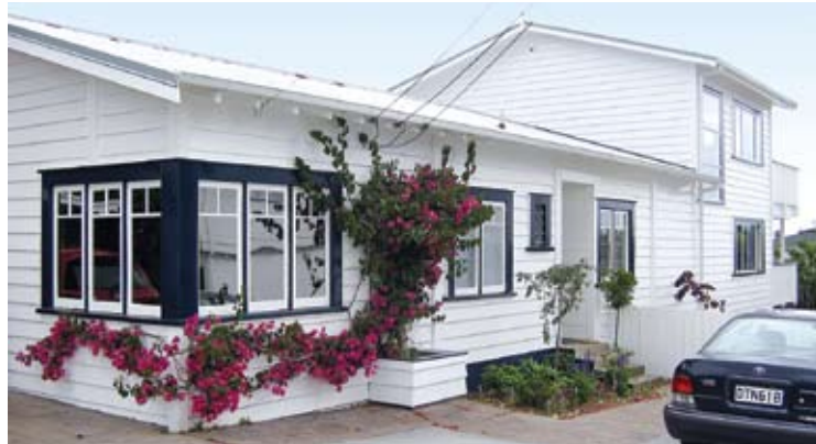
NEW HOME: The renewed bungalow with its two level addition.
